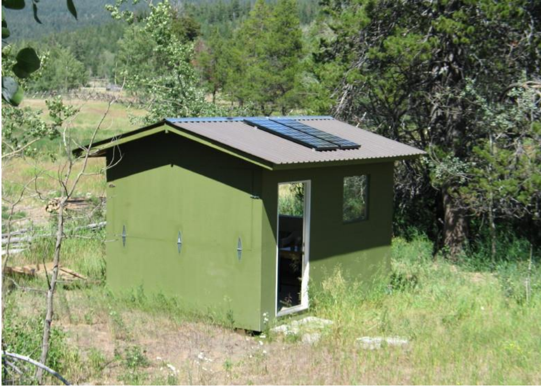
Figure 5. Banding station showing solar panels on roof.
