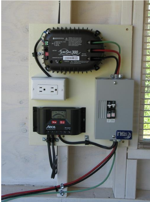
Figure 6. Solar power control system.
