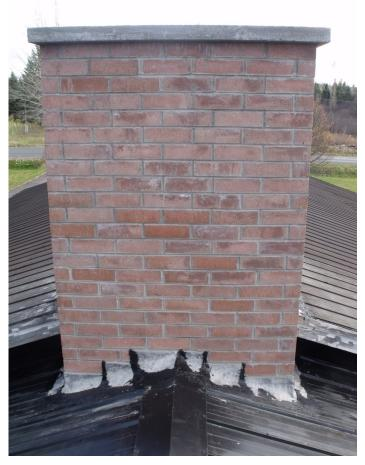
Artificial roost chimney constructed on a private garage in New Brunswick. The roost has not yet been used by swifts despite being similar in size and characteristics to a roost chimney in Bathurst that is used annually by large numbers of swifts. Photo: Lewnanny Richardson
